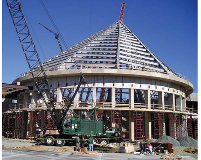
Construction continues on schedule for the 2006 opening of the National Museum of the Marine Corps.
