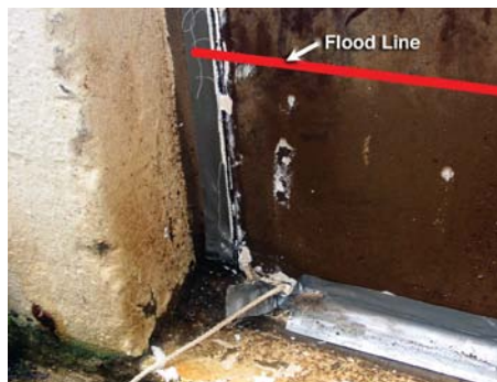
The basement door of Building 58 was sealed with tape and putty to keep out flood waters during the rainy season.
