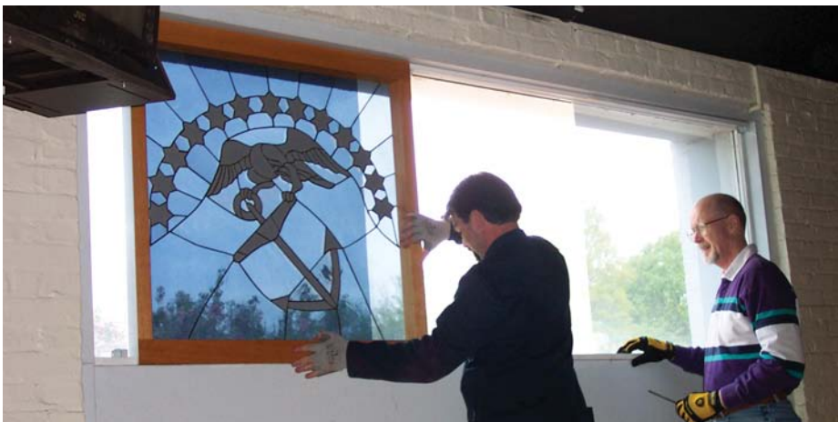
Museum staff members Ronnie Alexander and Gordon Hiem carefully remove the stained glass HD emblem from above the main entrance of Building 58 on the Washington Navy Yard in preparation for HD's move to Quantico, Virginia, in September.
